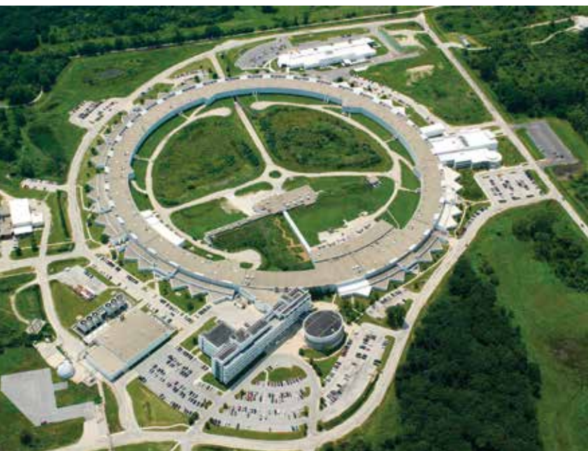
The intense X-ray facility—comprising the huge magnetic storage ring and dozens of individual beamlines for research—at Argonne National Laboratory that has enabled academic scientists to determine complex molecular structures and helped pharmaceutical scientists optimize new drug candidates for clinical trials. (Mark Lopez / Argonne National Laboratory)
