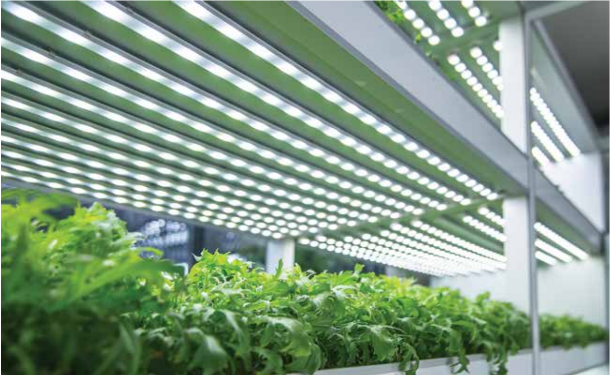
Semiconductor devices known as light-emitting diodes are not only very efficient, but can also be “tuned” to emit light of different colors for different purposes—“warm” white light for human residential use, or “cooler” white light that helps plants grow optimally for indoor agricultural use. ( Zhang Sheng / Shutterstock.com )
