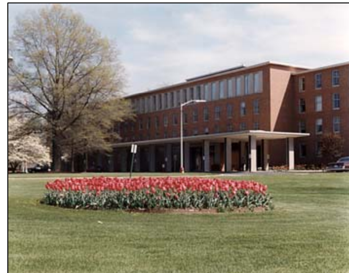
DOE Germantown Building, Germantown, MD
