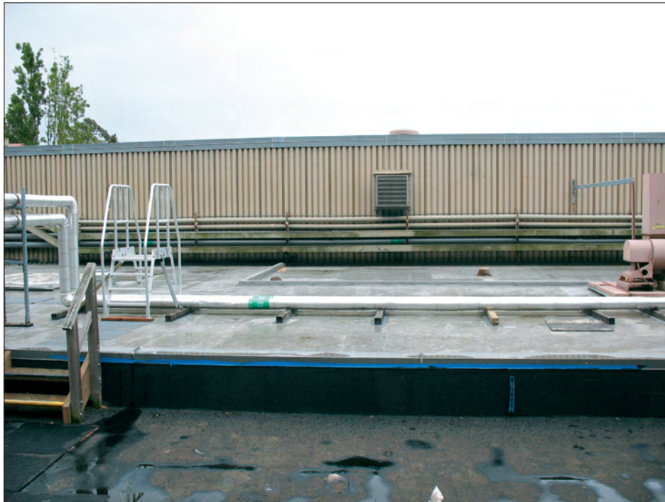
A. Building 71 roof area to be altered
