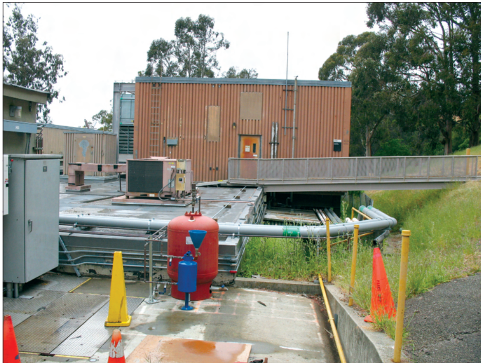
B. Building 71 roof area to west showing variety of existing roof structures
